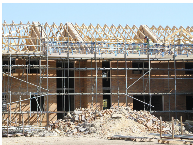
New Forest District Council homes under construction (2018).
