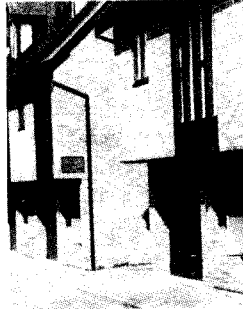
Neatly designed meter cupboards
