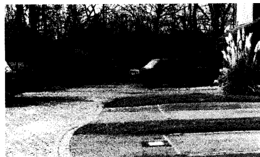
Establishment of a road system
