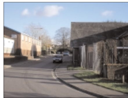
Unattractive rear of Avonway and Drill Hall
