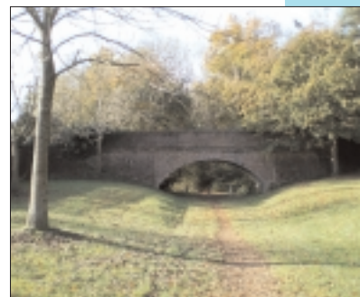
Old railway bridge
