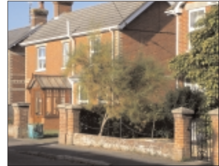
Walls in Alexandra Road
