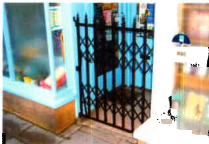
An iron gate can add security to a recessed entrance
