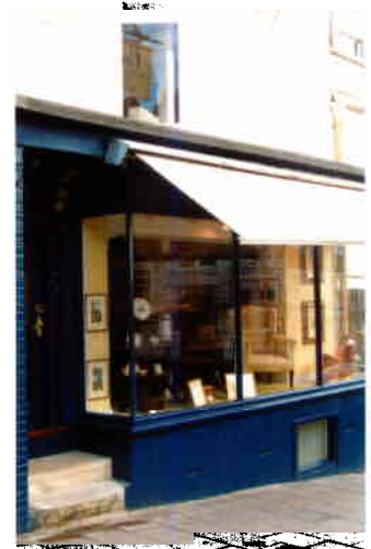
New blinds should be capable of being retracted into a recessed area
