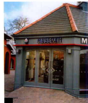
Combination doors are designed to continue the theme
