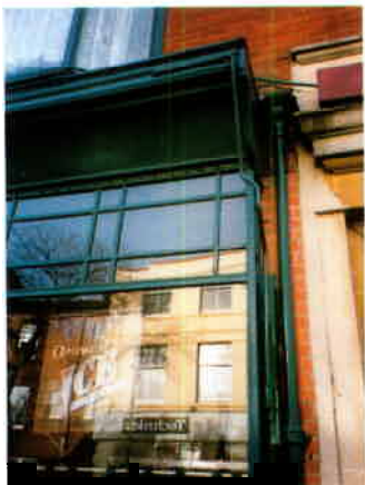
Large areas of glazing subdivided with a trellis of glazing bars
