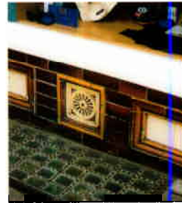
Glazed tiles and brickettes in stall riser.
