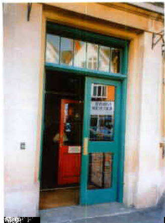
A high opening subdivided to incorporate traditional door heights with a well proportioned top light above
