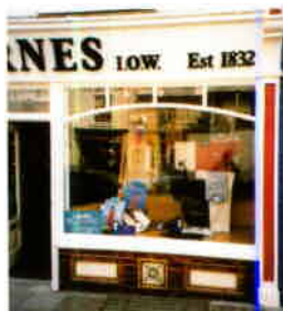
Simple Edwardian style with a shaped head over a glazed tile base
