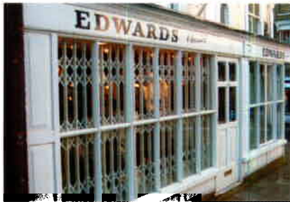
A mesh security screen allows displays to be viewed after trading hours
