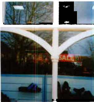
Shaping achieved by joining mullion and transom with a curved bracket
