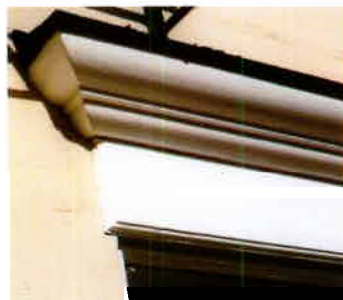
A simple fascia and cornice projection
