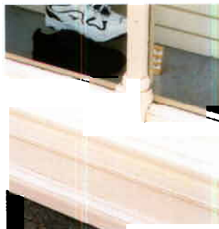
Rounded mullion onto a square stooling
