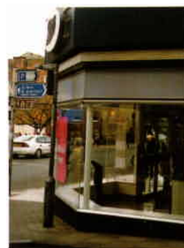
60's style. A cumbersome fascia with little support looks very top heavy
