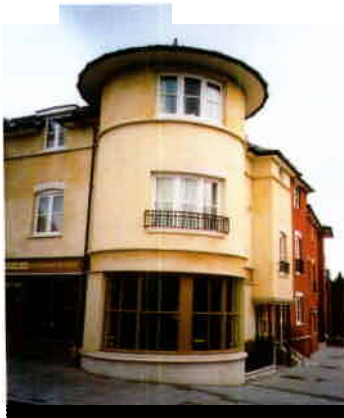
This new development has been designed to emphasise a quality commercial frontage at ground level and complement the locality
