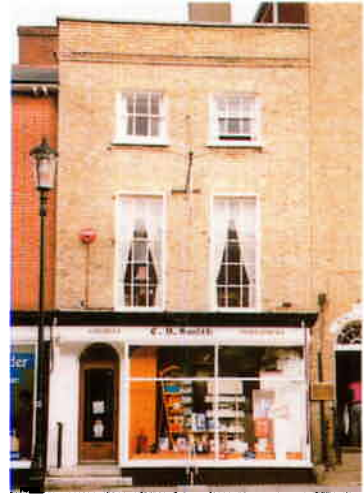
Large sheets of glass and low windows are vulnerable
