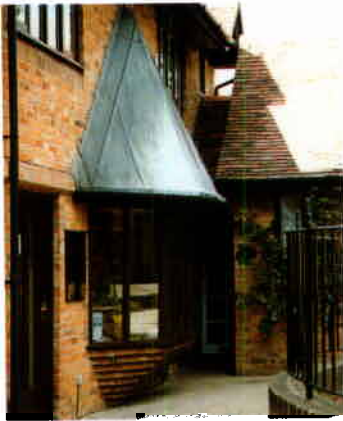
A corbelled bay with vertical panes under a lead roof
