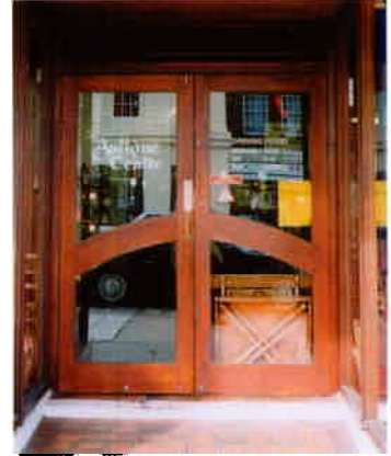
The centre rail reflects the style of a curved window
