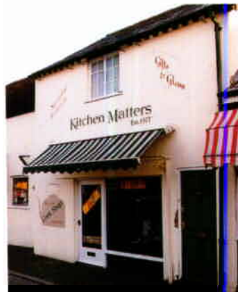
A modest scheme which introduces a blind and painted signs on the elevation
