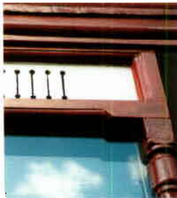
Stylised slots vent the area above the window
