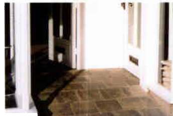
Riven slate takes up changes in level
