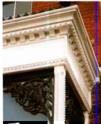
The cornice consists of several rounded profiles above a dentil course
