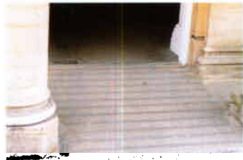
Carborundum strips set into stone aggregate screed
