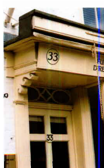
Fascia continues over doorway, supported by a shaped bracket,
