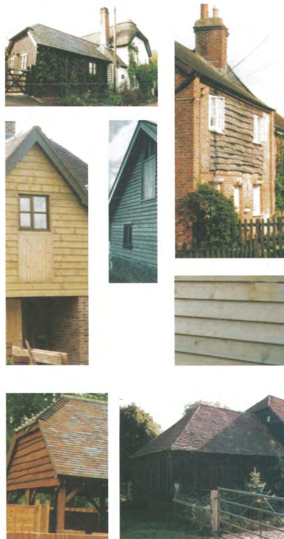
Use of both horizontal and vertical cladding ▲
