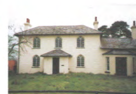
Masonry paint on render
