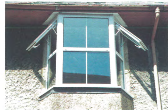
Non-traditional materials, weak sections and cumbersome fanlights ▲
