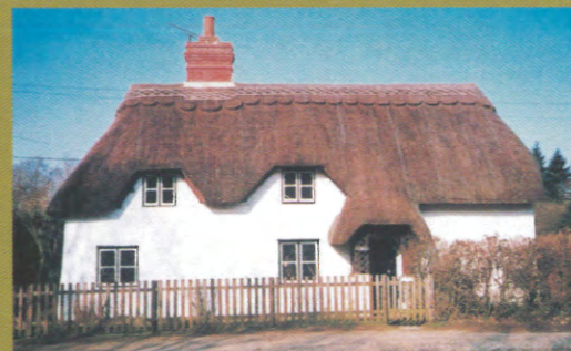
One and a half storey cottage with rendered finish and thatched roof
