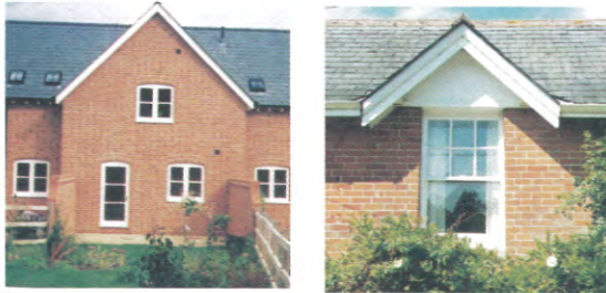
Casement (left) and Sash (right) windows ▲
