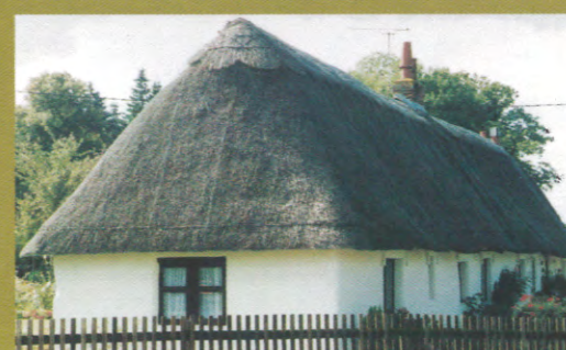
Single storey cob cottage of long narrow proportions behind a picket fence
