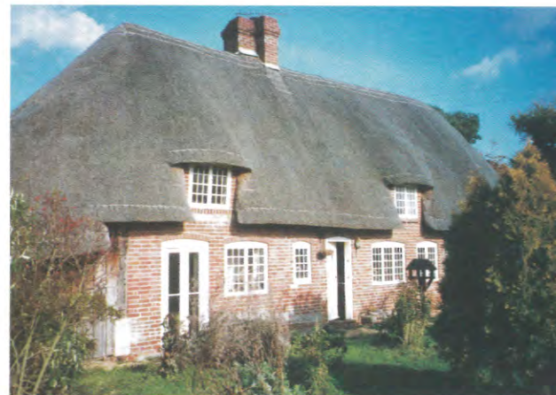
Longstraw thatch at Breamore - note the simple ridge ▲
