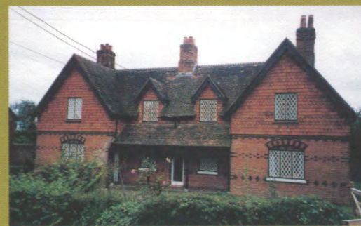
Estate cottages utilising a range of materials - patterned brick, tile hanging, clay tiled roof and cast iron windows
