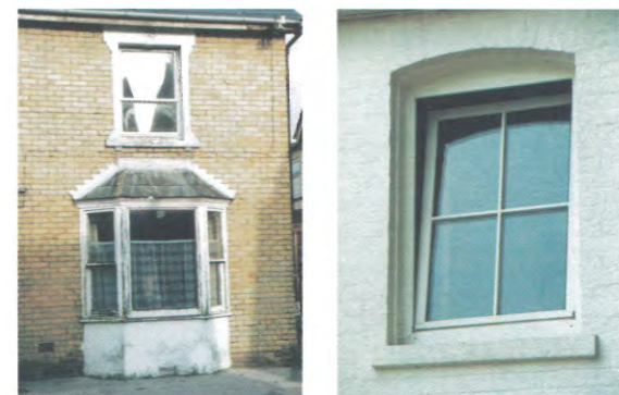
The effect of missing glazing bars (left) and awkward looking tilting windows (right) ▲
