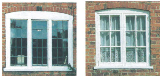
Balanced, flush framed casements with centre bar (left) and '8 over 8' sash (right) windows ▲
