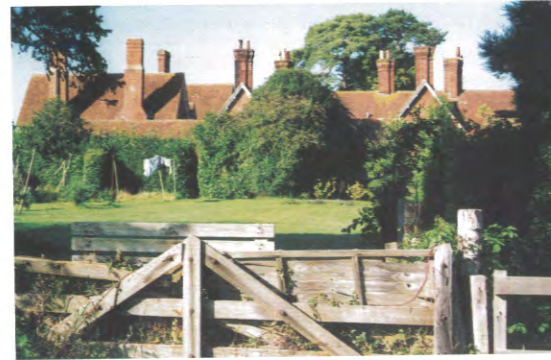
Historic peg tiles, Beaulieu
