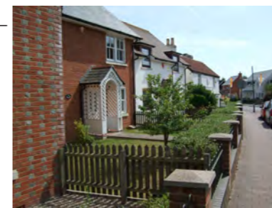
Domestic and rural scale dwellings define the east side of the old village green.
