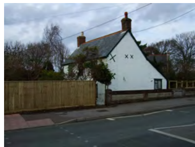
Remnant of the rural past. A single older forest cottage, its cat-slide roof form, retained window proportions and its position against the street is significant in the street scene.
