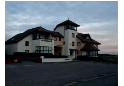
Distinct 'stop end' where the skyline rises to a three-storey landmark at Greenside Court.
