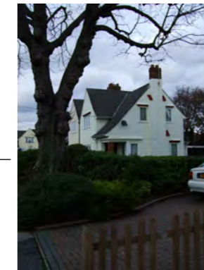
Cul-de-sac at Peckham Avenue where distinct sets of similar dwellings create their own identity within the wider neighbourhood. All of similarly rendered finish with characteristic gables under steeply pitched roofs. They vary only by colour. Beautifully proportioned, these simple forms with modest detailing rely upon gardens to offer up variety and further decoration. The original pairs are marked, later bungalow infill picks up some of their character.
