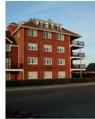
Occasionally taller buildings are situated near the central arrival point.
