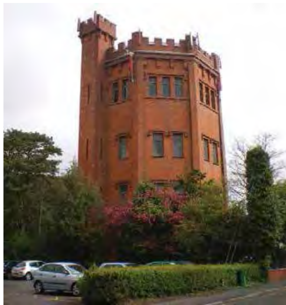
Figure 3 - The Water Tower
