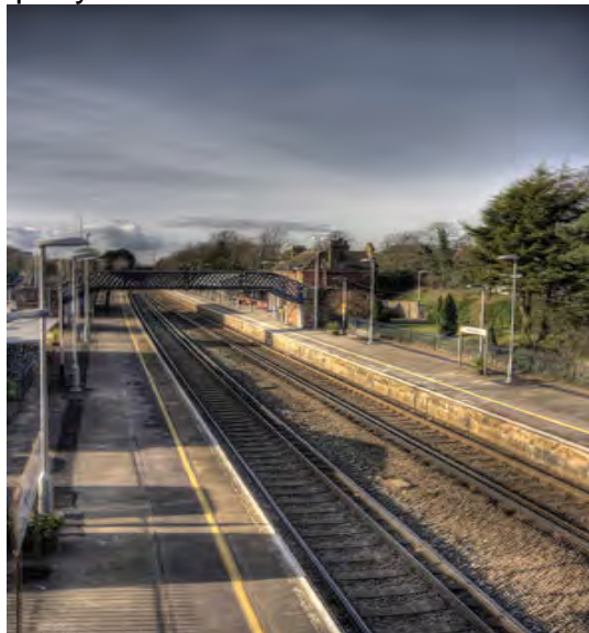
Figure 2 - New Milton Railway Station
