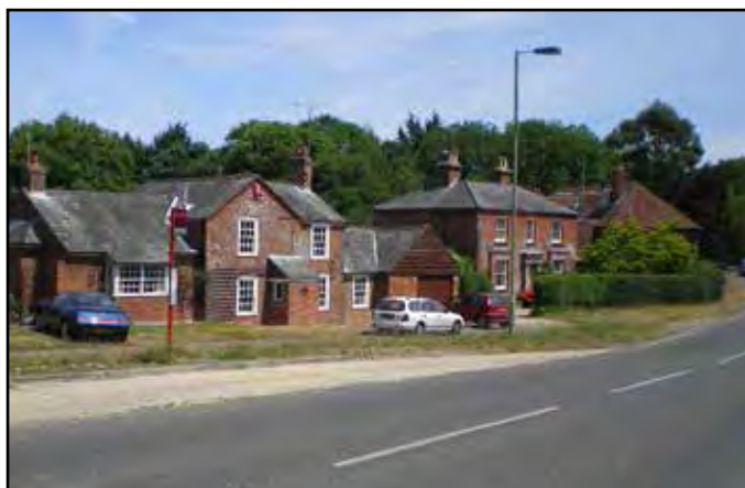
Mill cottages and Grade II Listed Mill at Efford
