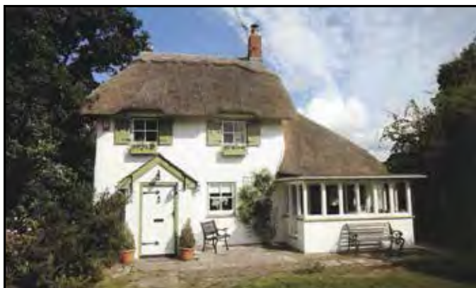
Swan Cottage-(formerly Yeovilton Lodge and Everton Post Office) a traditional cob cottage (Listed grade II) *5
