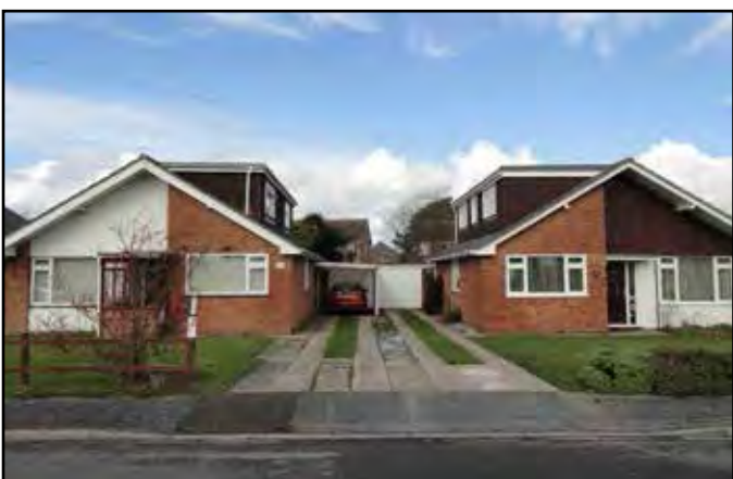
Impact of roof conversion at Pinewood Estate
