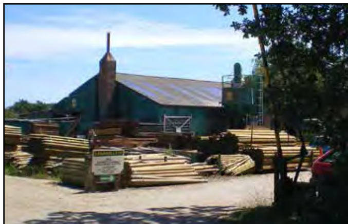
Construction & building materials business Crabswood Lane
