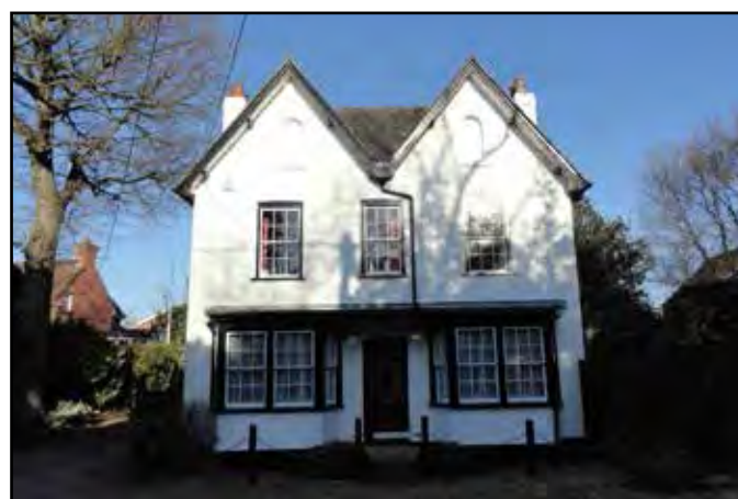
Rodbourne House, an early building on Christchurch Road
