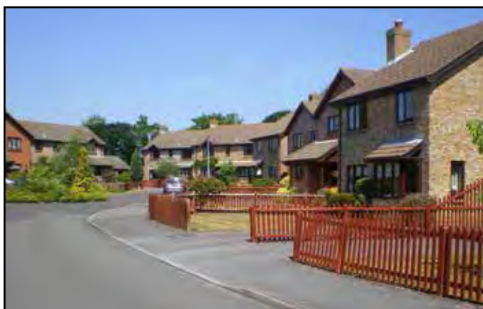
Brickwork and limited landscape at Laburnham Drive
