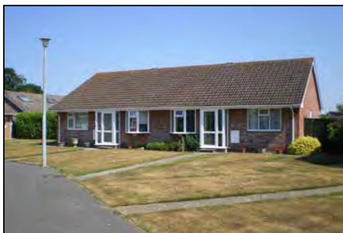
Minimal landscape to bungalows at Rodbourne Close
