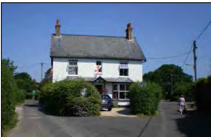
The former Post Office at the junction of Centre/East Lanes
