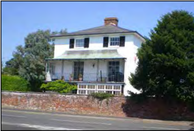
Yeovilton House is one of the Listed Buildings in Everton
