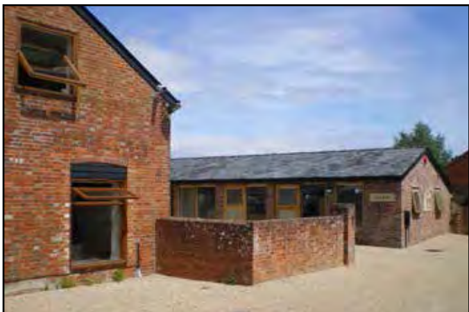
Office development at Efford Farm
