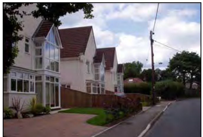
Overbearing development in Stopples Lane
