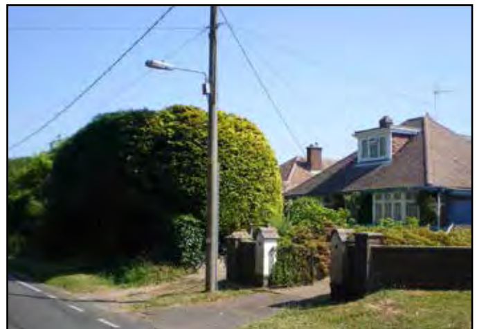
Impact of overhead cables
