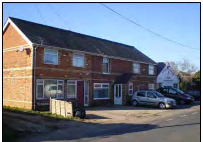
Impact of extension of cottage next to Tiptoe Garage
