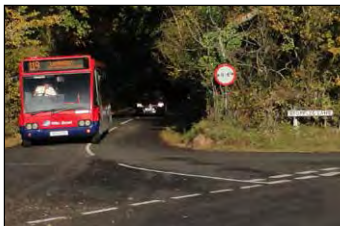
The sharp turn at the Stopples Lane/Hordle Lane Junction
