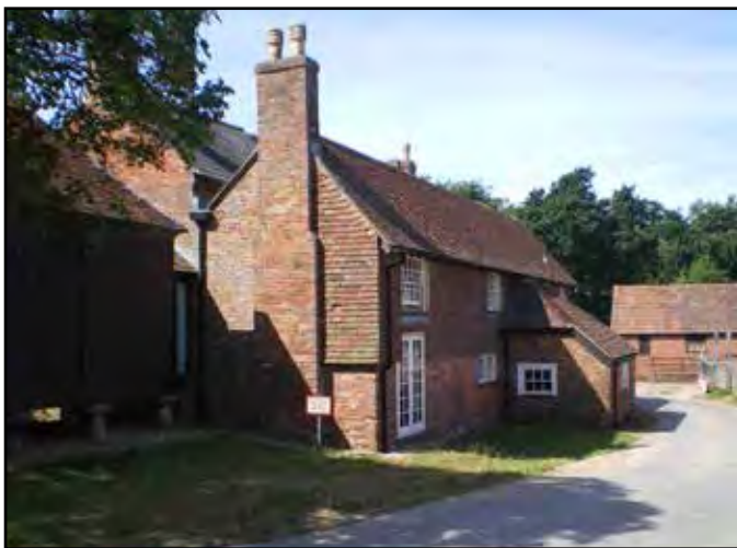
Listed buildings at Leagreen Farm
