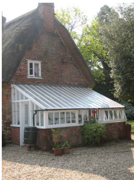
This glass "orangery" complements the cottage
