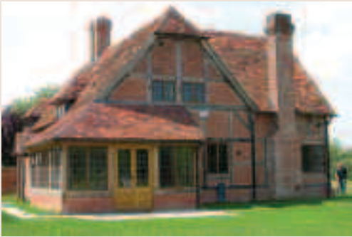
A hipped clay tile roof which reflects the character of the original building is used to good effect.
