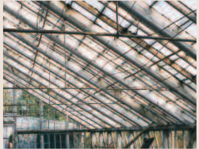
Historic conservatories and glass houses often have structural delicacy and finesse.
