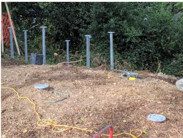
Figure 31. Less invasive screw piles being installed inside the RPA's of protected trees to support new structures
