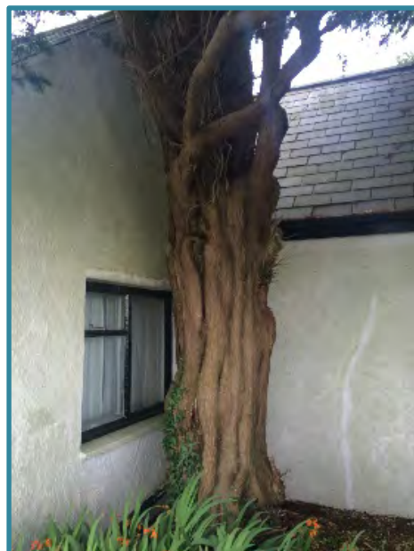
Figure 9. A mature Yew tree situated in close proximity to the dwelling
