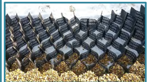
Figure 11. A cellular confinement system awaiting infill
