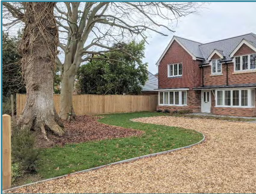
Figure 12. A new access and driveway situated in close proximity to protected, mature Oak and Beech trees through the use of a 3D cellular confinement-based surfacing system
