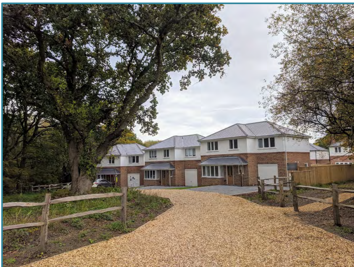
Figure 1. A mature Oak tree successfully retained in a newly completed development
