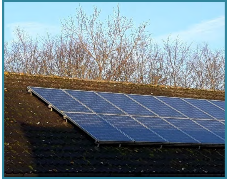
Solar panel shading
