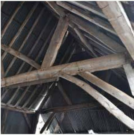
◀ This timber roof is failing and repairs are needed to maintain the integrity of the structure
