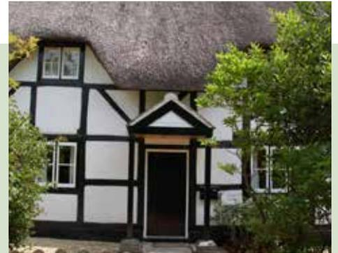
Example of timber frame with painted brick infill panels
