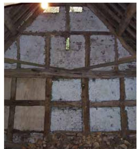
Irregular shaped crevices can be packed with lime hair plaster and lime washed over
