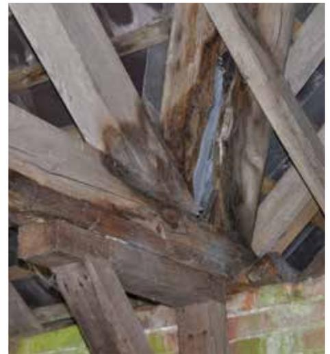
These structural timbers have started to rot as a result of a leaking roof
