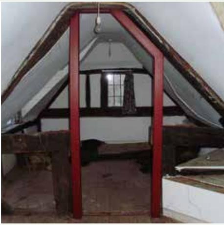
◀ Cutting a doorway through the collar of this roof is not recommended as it could seriously weaken the structure of this timber framed cottage and leads to loss of original historic fabric
