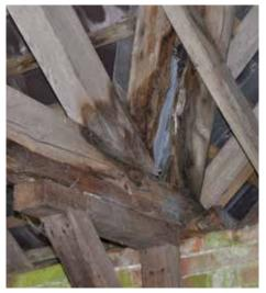
These structural timbers have started to rot as a result of a leaking roof
