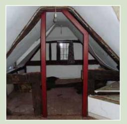
Cutting a doorway through the collar of this roof is not recommended as it could seriously weaken the structure of this timber framed cottage and leads to loss of original historic fabric
