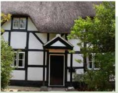
Example of timber frame with painted brick infill panels
