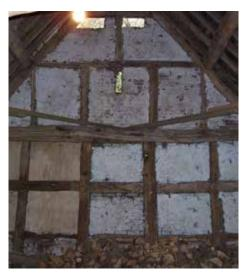
Irregular shaped crevices can be packed with lime hair plaster and lime washed over
