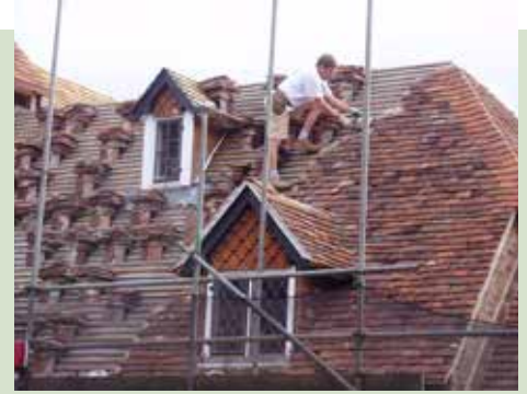
Tiling in progress
