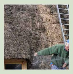
Patch repairs to a combed wheat reed roof
