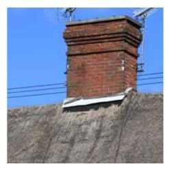
Thatch around the chimney is badly eroded
