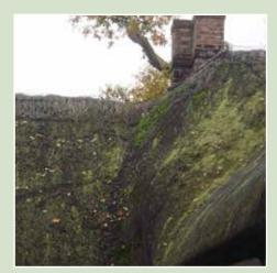
Moss build up on a deteriorating thatched roof
