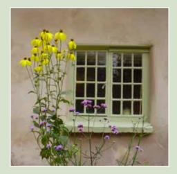
Limewash is the preferred finish on traditional buildings as it allows the structure to breathe, enabling damp to evaporate away rather than being trapped in the wall
