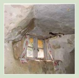
This patched ceiling and wall plaster continues to be affected by damp, as the cause of the problem has not
