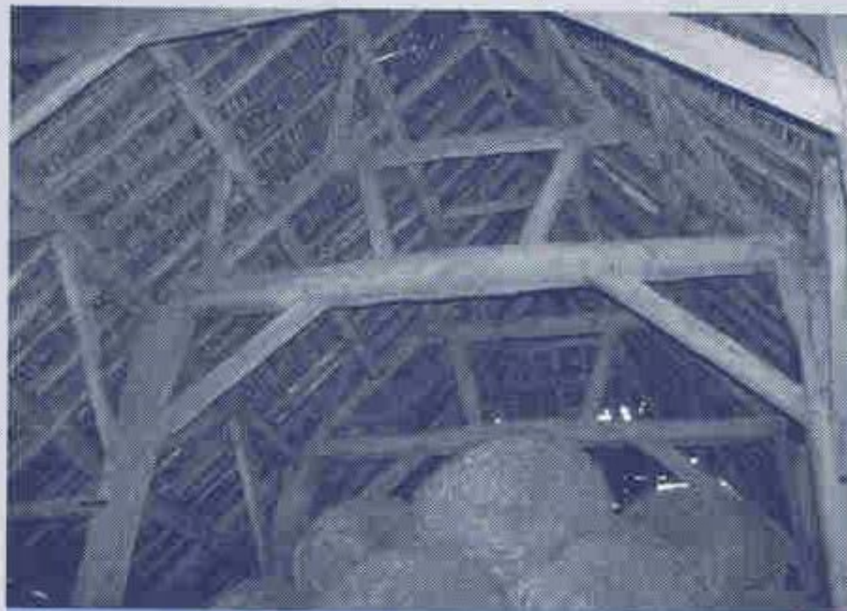
17th century timber framed barn
