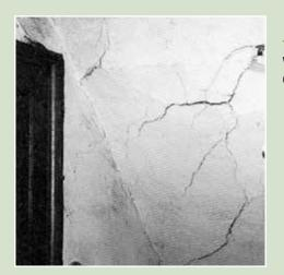
Wall plaster determines internal character. Old lime plaster on laths can be repaired
