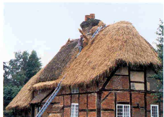
Thatch receiving top coat
