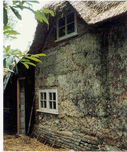
Clay Cob cottage showing layers
