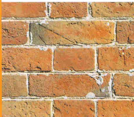
C19th brickwork in lime mortar
