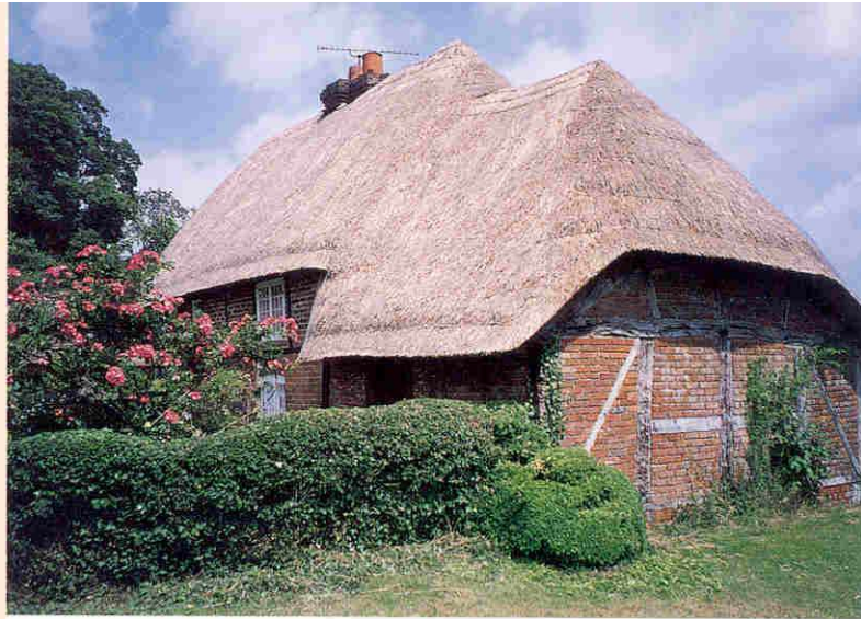
Traditional long straw thatch with flush ridge
