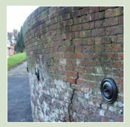
This wall was leaning badly, but has been stabilised using steel rods tied to ground anchors. The method was less invasive than having to completely rebuild the wall
