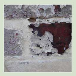
Plastic paint does not allow the brickwork to breathe, trapping moisture in the wall
