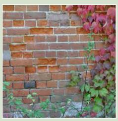
Where cement mortar pointing has been used and is noticeably resulting in the spalling of the faces of the bricks, it should be assessed whether it can be readily removed using non-mechanical tools.
