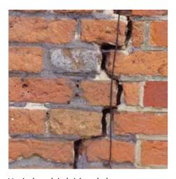
Vertical crack in brickwork due to movement. Brickwork has been repaired with a variety of hard mortars which have failed to address the problems
