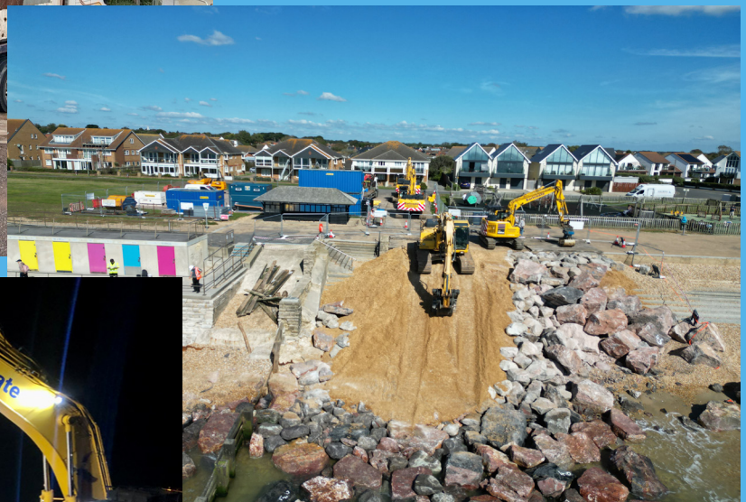
Temporary access to beach
