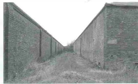
Walls around Magazine C
