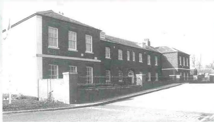
Barrack block, now converted to apartments
