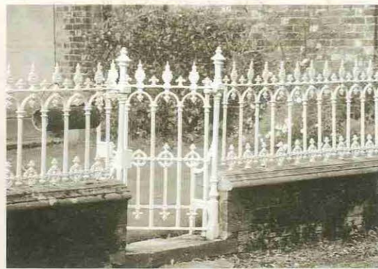
Listed railings at Nippard's Farm
