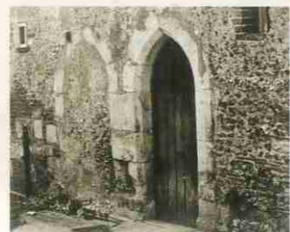
Old doorways at Manor Farm Barn
