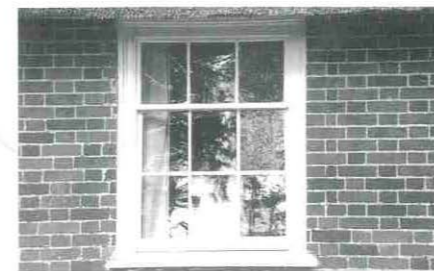
Old glass is an important feature and should be retained
