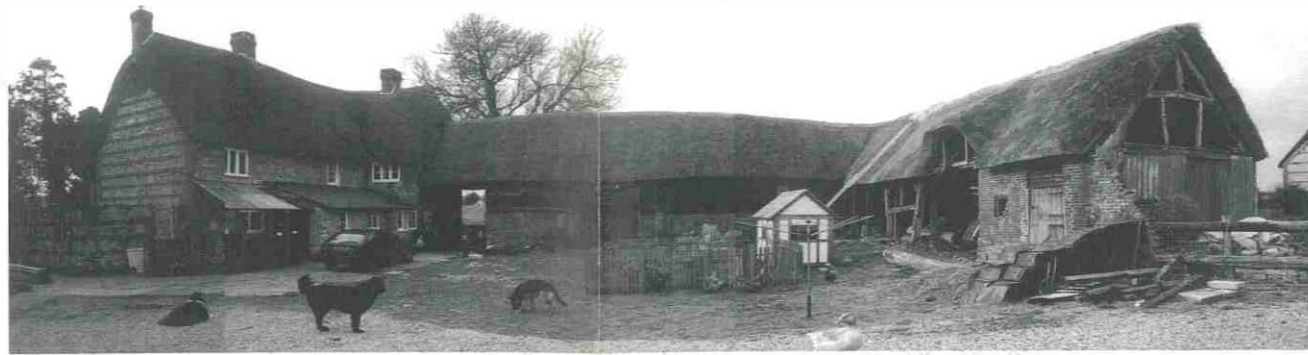
Talk's Farm - now almost completely repaired
