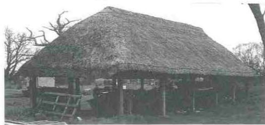
Cartshed, Harbridge Farm
