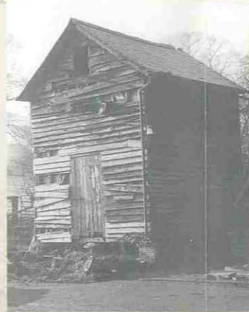
Timber staddle granary
