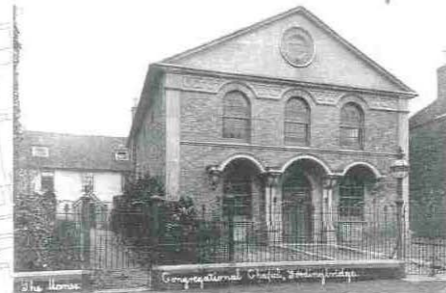
The loss of the railings has radically altered the street scene today
