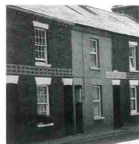
Original and altered unlisted terrace houses
