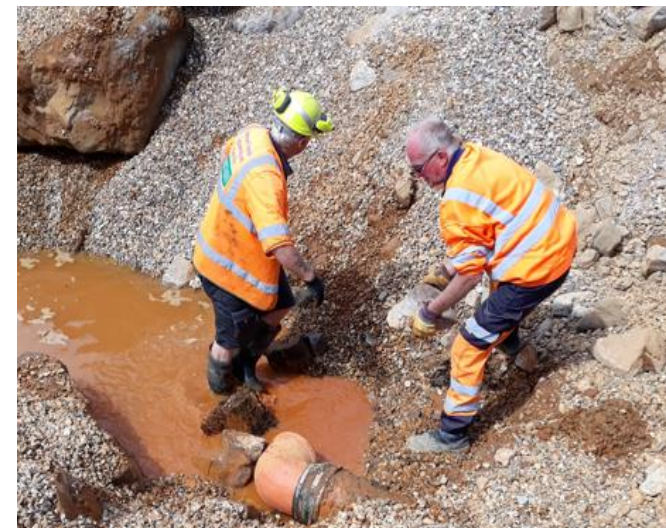
Maintenance of outfalls
