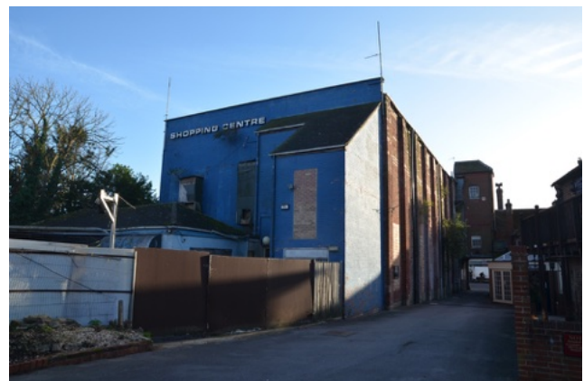
Figure 55: Rear view of 2 Market Place which is unsympathetically extended and repurposed, neglecting its historical value
