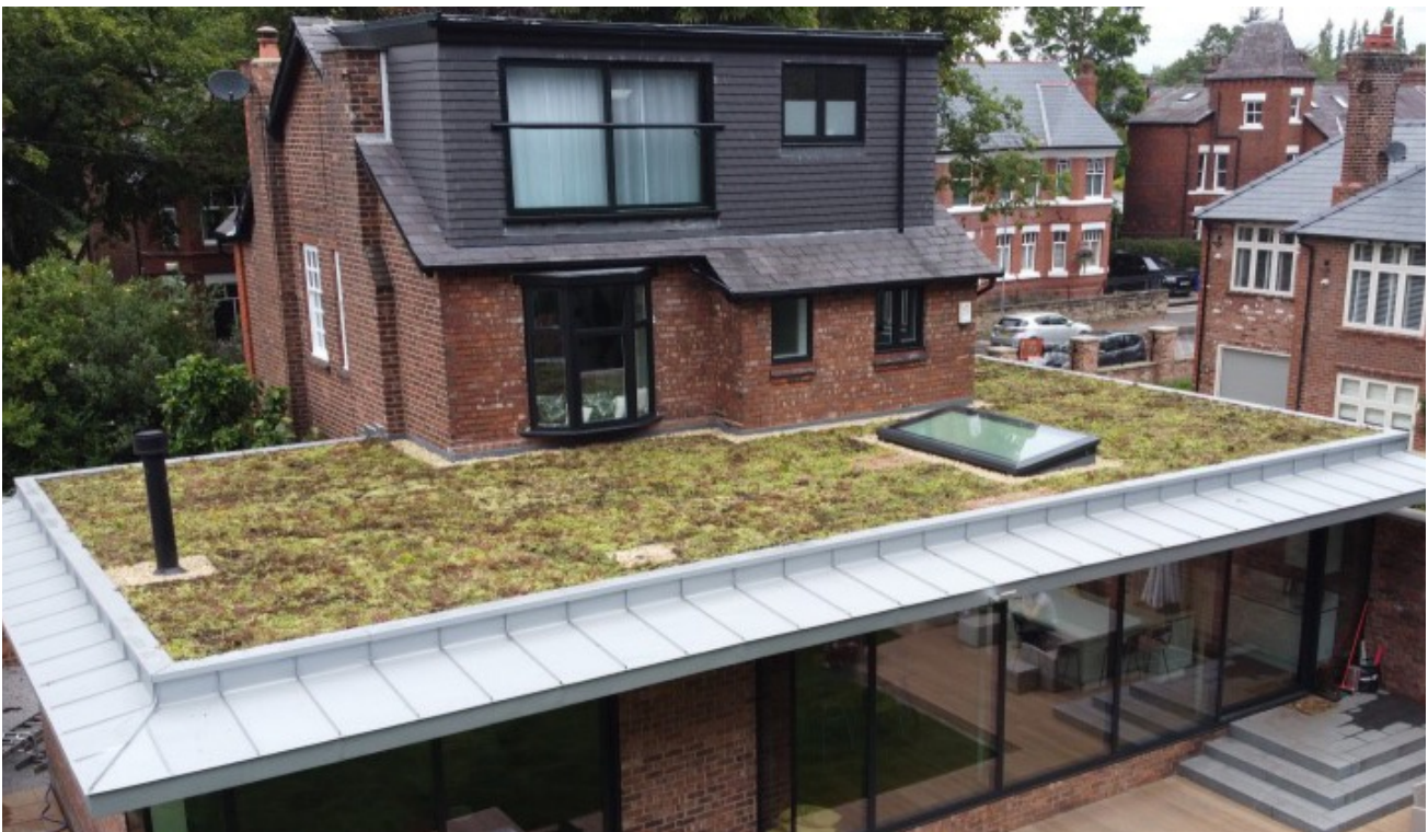
Figure 70: Lightweight green roof on residence in Manchester, UK (Source: https://www.sempergreen.com/en/references/private-residence-1 ).
