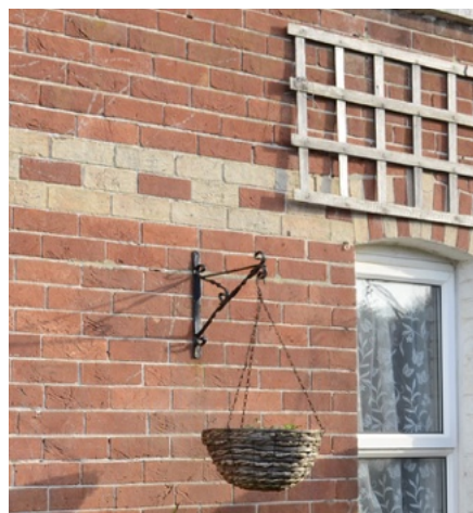
Fascia in buff alternated with red bricks
