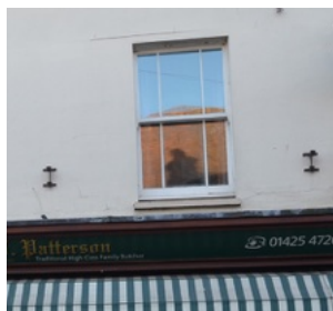
Sash window with rendered wall
