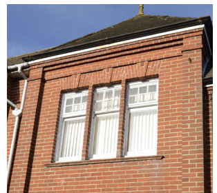
Sash window with brickwork
