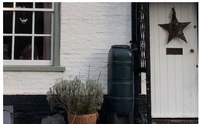
Figure 72: Examples of water butts used for rainwater harvesting.
