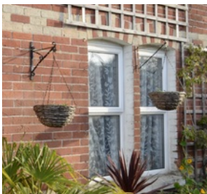
Casement window with some yellow brickwork around
