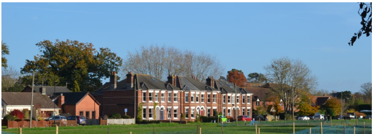
Figure 52: The subtle variation in the eaves and ridge levels create a harmonious roofline that is well integrated with the vegetation and countryside in the background.
