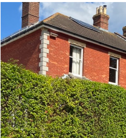
Red bricks building with white cornerstone and inlets stone used as windows details
