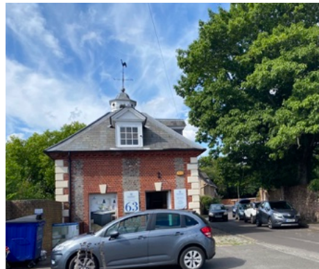
Red bricks building with white cornerstone and inlets stone used as windows details
