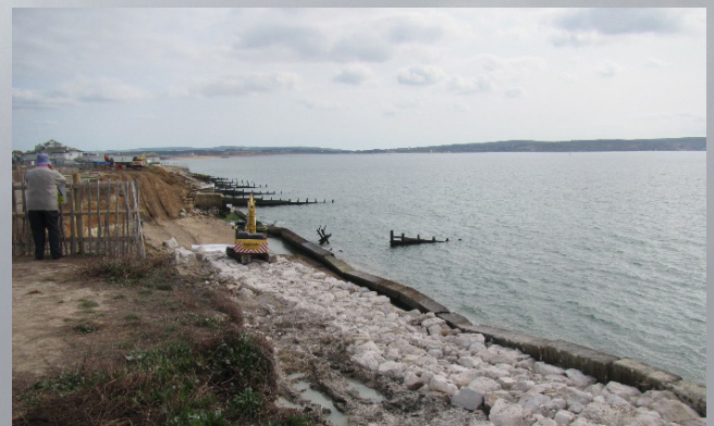
Constructing the "roadway" for the revetment
