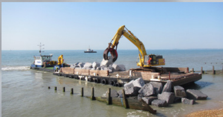
Unloading the rock for the new revetment
