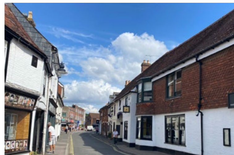
4. Lower end of Southampton road
