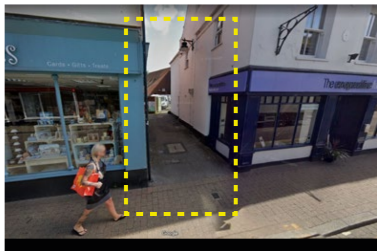
5. View from High Street to Northumberland Court
