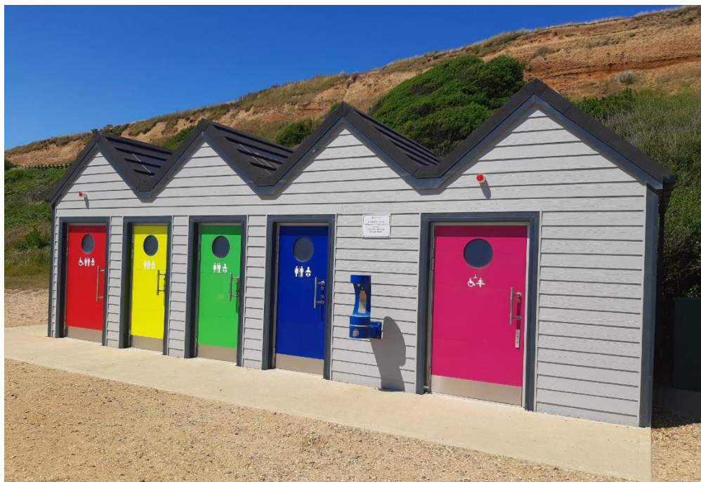
Barton Beach Public Toilets
