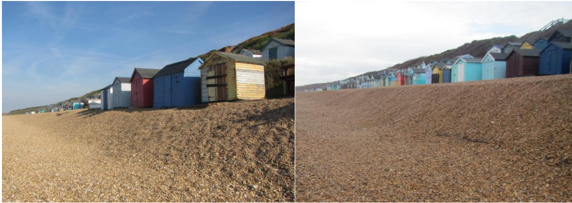
General arrangement of beach huts (2 rows: one on the beach and one on the lower cliff)
