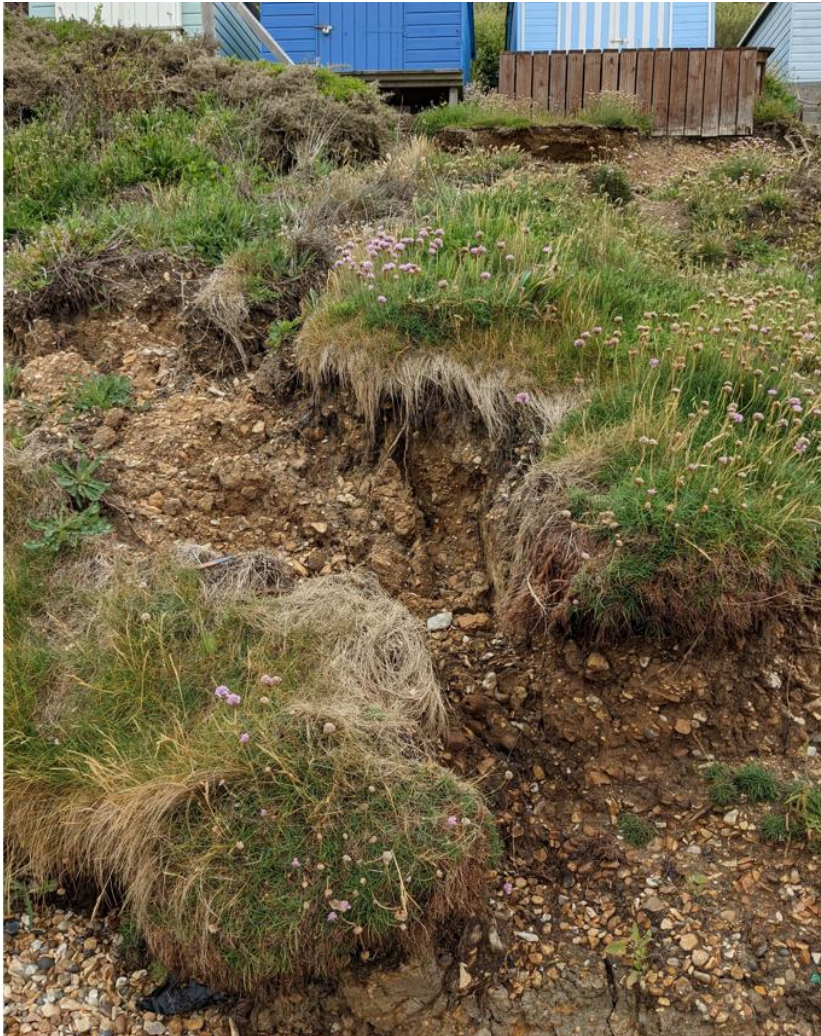
Figure 0-15 Photo of the slumped material at the western cliff slump. Photo taken 07/06/2022. Approx. Ordnance Survey grid reference SZ 27708 91760.
