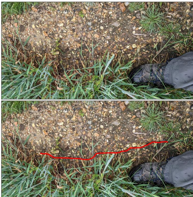
Figure 0-10 Photo of crack, taken 07/06/2022. Approx. Ordnance Survey grid reference SZ 27720 91763.
