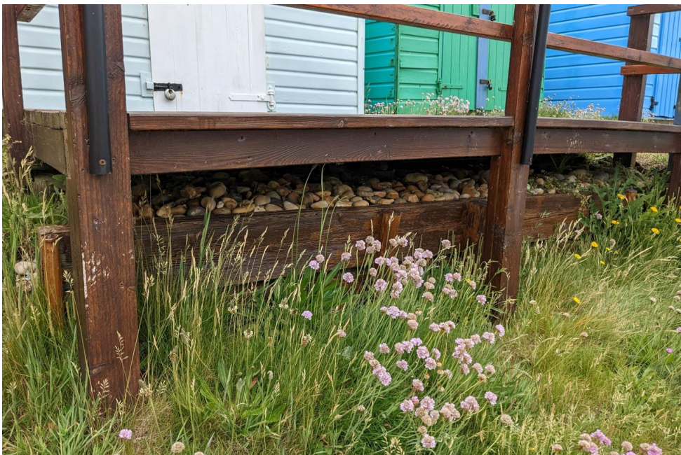
Figure 0-3 Example of ground raised and retained for beach hut and decking placement. Photo taken on 07/06/2022. Approx. Ordnance Survey grid reference SZ 27702 91768.
