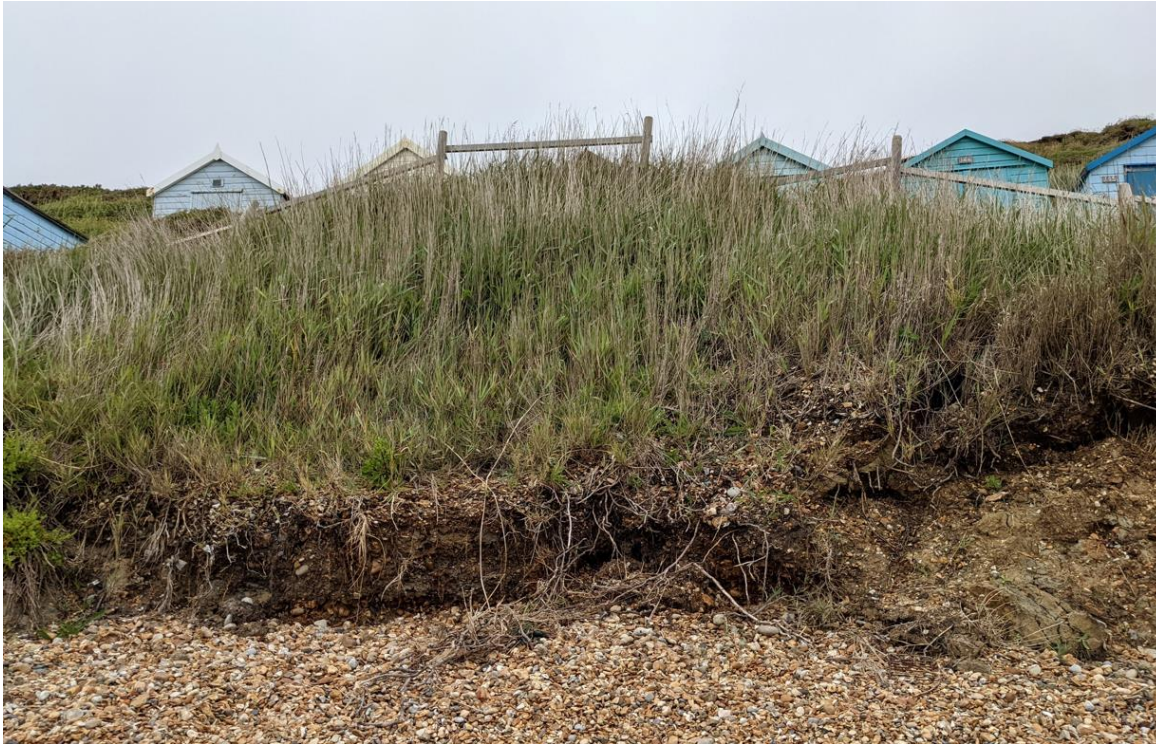
Figure 0-22 Photo of unsupported toe of the slope in the middle cliff slump area. Photo taken 07/06/2022. Approx. Ordnance Survey grid reference SZ 27730 91751.
