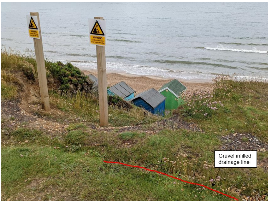
Figure 0-21 Photo of failure at the top of the cliff, adjacent to the drainage channel, taken 07/06/2022. Approx. Ordnance Survey grid reference SZ 27649 91814.
