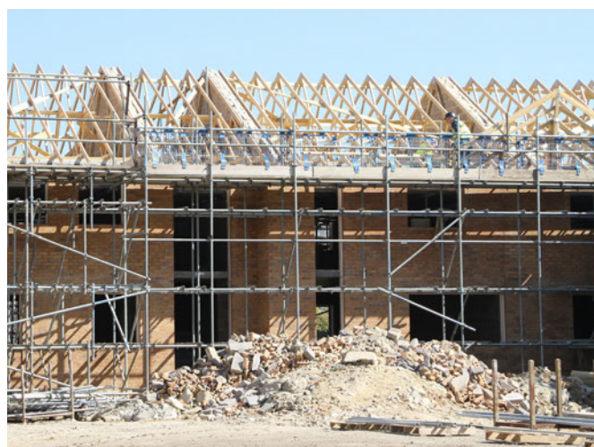
New Forest District Council homes under construction (2018).
