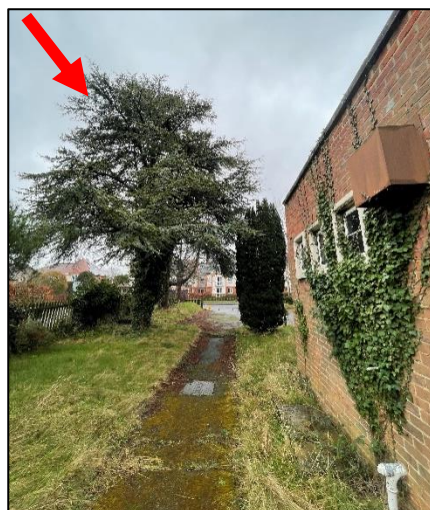
Photograph 6: View of tree T9 from western vantage within site (1 st March 2022), highlighting the proximity of the tree to the existing building.
