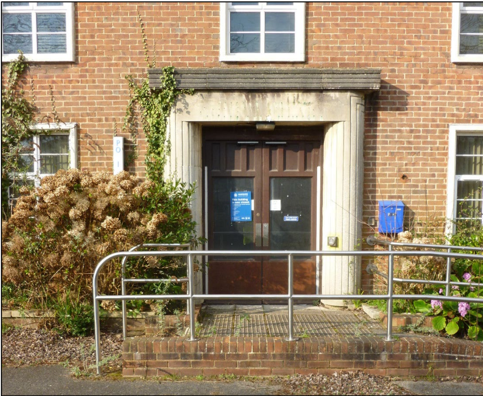
Plate 9: The Police Station's front doorway
