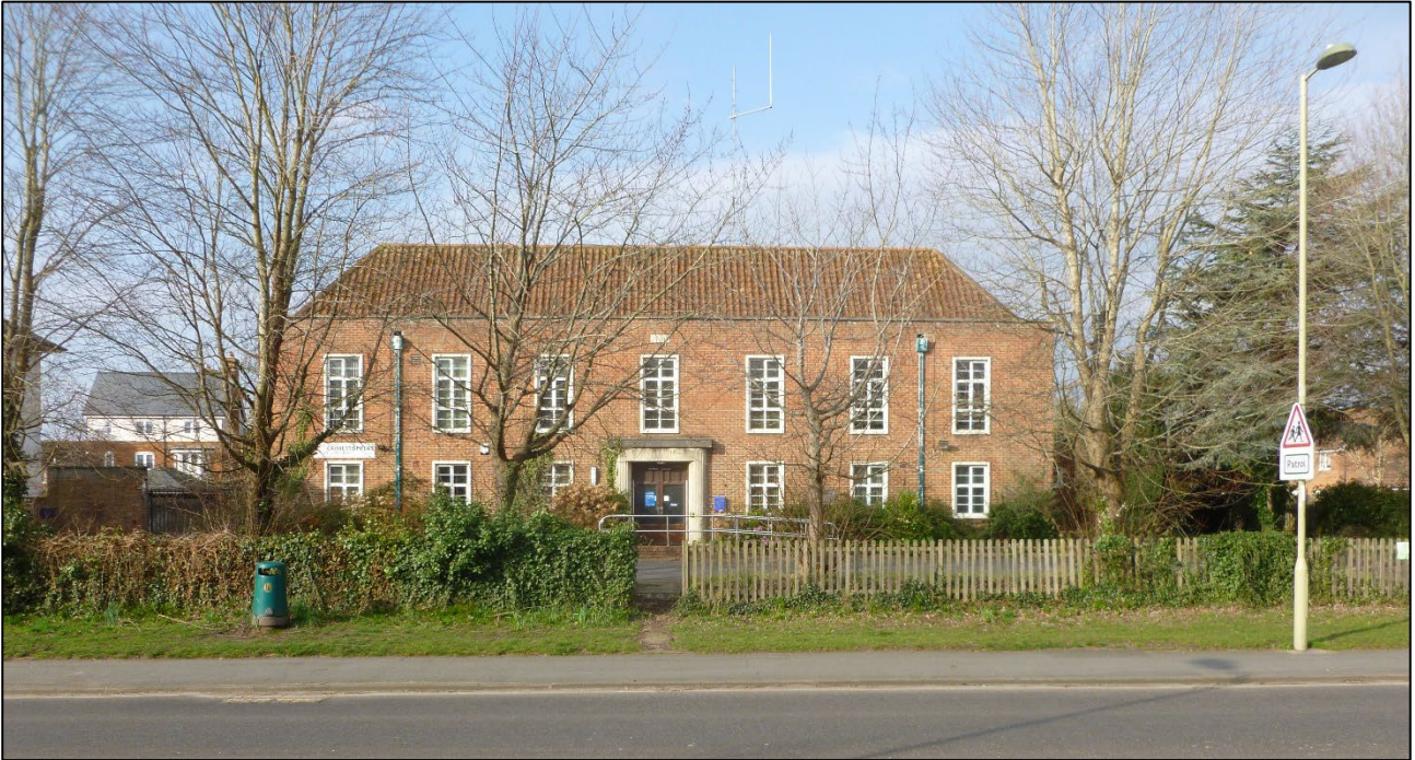
Plate 1: Main elevation, eastern, of Lymington Police Station from Southampton Road
