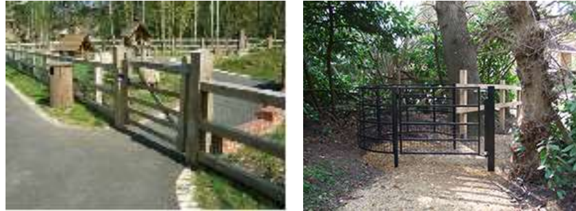
Examples of typical accessible barriers
