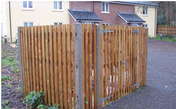
A communal store screened from the surrounding open space.
