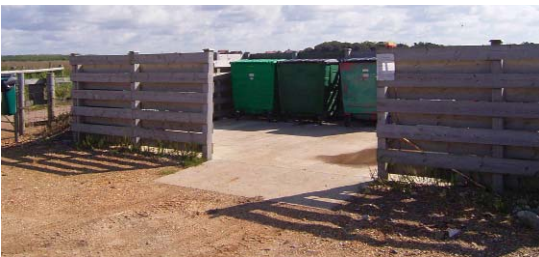
Additional storage for bins suitably designed to relate well to the open rural setting of a caravan park.
