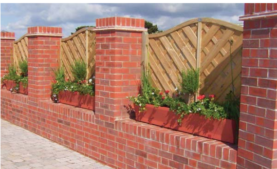
Here thought has been given to providing a well screened, accessible store for recycling and waste bins.
