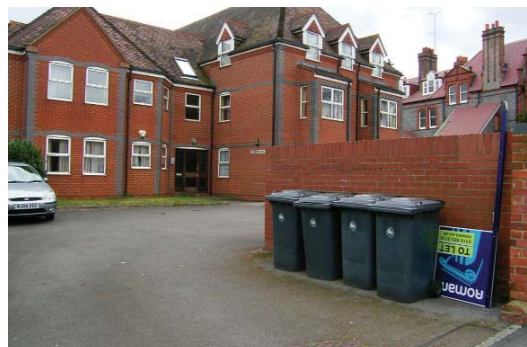
Not really what you want to see at the principal entrance to a block of flats.
