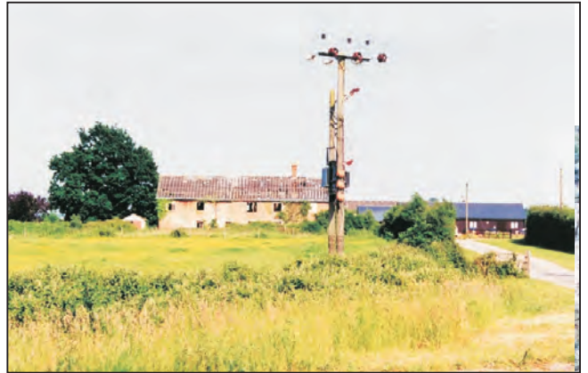
Dereliction of traditional buildings
