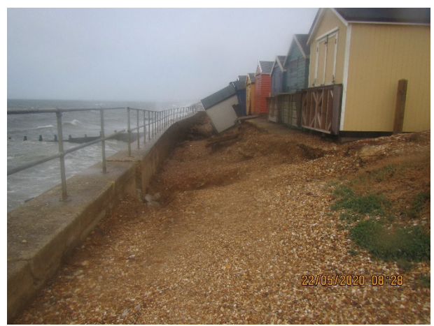
27 February 2020 and 22 May 2020 - Beach huts falling forwards into the void in Area 2.
